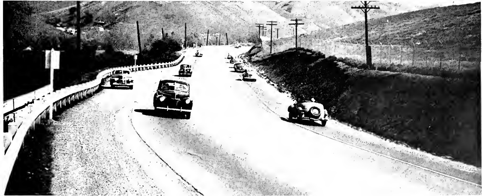
Three busy sections of U. S. 40 recently transformed from a three-lane to a four-lane highway
